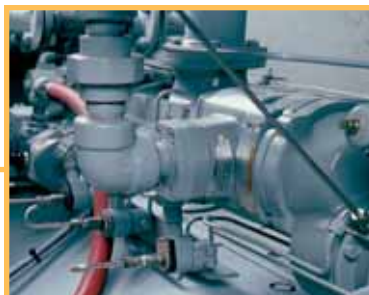
The ST799GCDP03R31 starter is piped for use with gas on a Waukesha F3521GU used for power generation.
